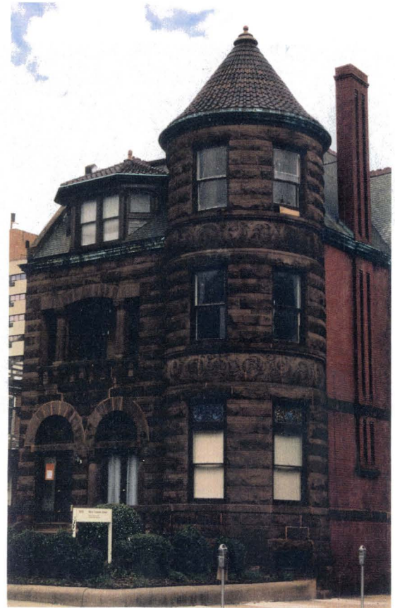
Figure 22. 1000 West Franklin Street. (Photo: Author)
