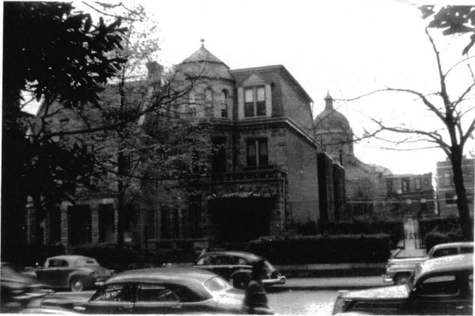
Figure 12. Barksdale House, 813 West Franklin Street. Built ca. 1887; demolished 1950s. ( James Branch Cabell Special Collections )
