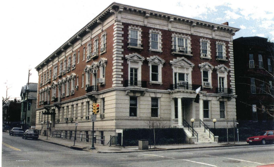
Figure 29. The Raleigh Building, 1001 West Franklin Street. Aubrey Chesterman, architect, 1907. (Photo: Author)
