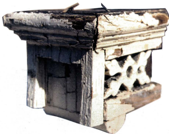
Figure 39. Modillion block from cornice of Bowe House, 917 West Franklin Street, 1887-1888. (Photo: Chris Dunham)
