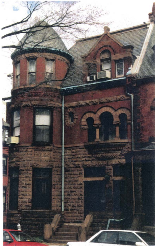
Figure 23. 924-930 West Franklin Street. (Photo: Author)
