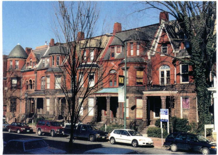
Figure 24. 932 West Franklin Street. (Photo: Author)
