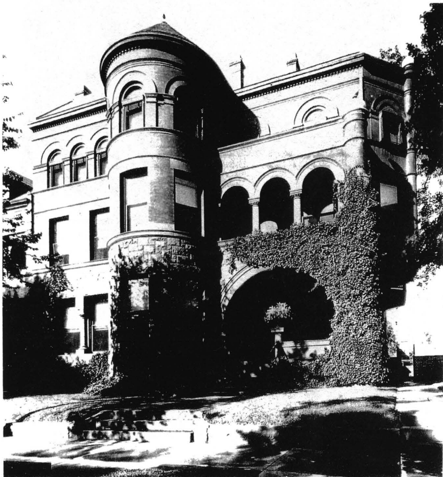
Figure 9. Hirsh-Williams House, 824 West Franklin Street. William M. Poindexter, architect, 1889-91; demolished 1937. ( The Valentine Museum )
